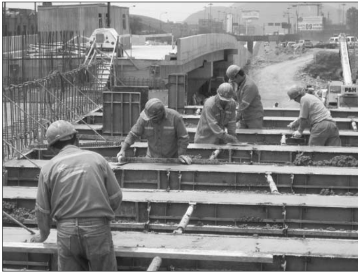
Workers complete one of several underground busways into Lima's Central Station, the core of the new system. - Photos for this article by Tom Rickert
